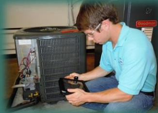
Heating, AC & Refrigeration
